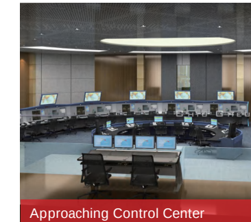
Approaching Control Center
