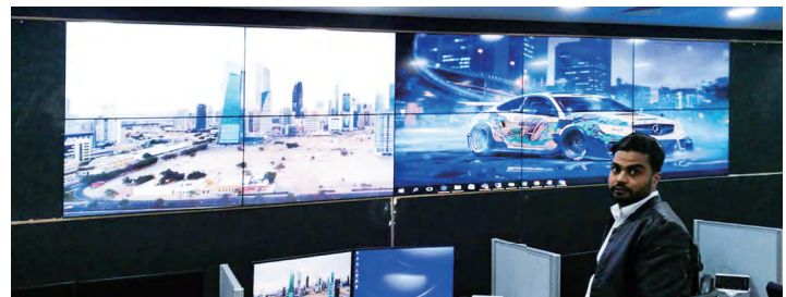
Network Operation Center(NOC) for National Bank of Kuwait
